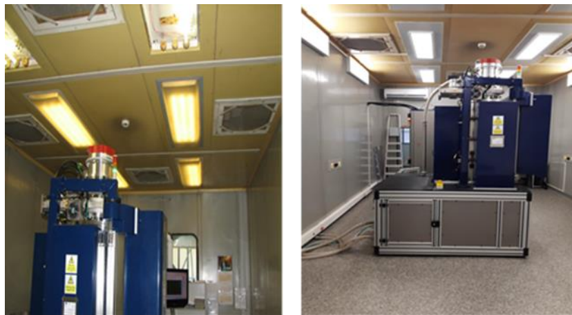
Photos of a technological room in the existing clean room, before (left) and after (right) the renovation.
